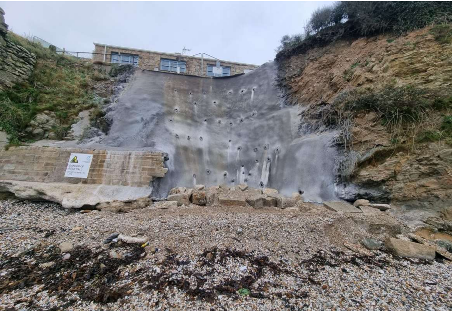
Pictured above: Completed stabilisation works.
