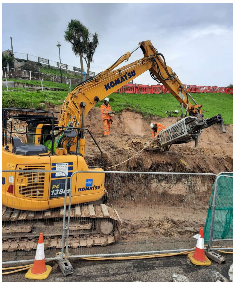
Pictured above: Griffiths rope access technicians installing soil nails with a 13t Zero tail swing excavator fitted with a hydraulic drill mast
