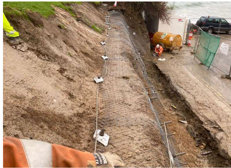
Pictured above: Fig 1) Griffiths rope access technician installing soil nails. Fig 2) Griffiths rope access technicians attaching spike plates post installation of soil nails. Fig 3) Completed slope stabilisation.
