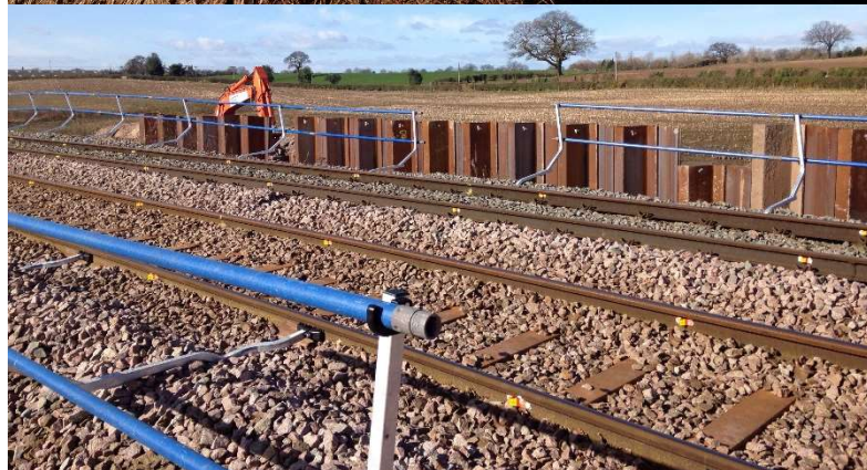
Fig 1) Train running on embankment whilst sheet piles are being installed.
