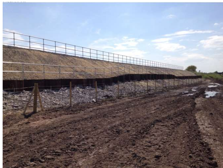
Pictured above: Fig 3) Original track defect with significant loss of geometry. Fig 4) Drilling works with 36T excavator on crest and 13T excavator on the toe. Fig 5) Completed sheet pile on one side of railway with regrade, safe cess, handrails and fencing.
