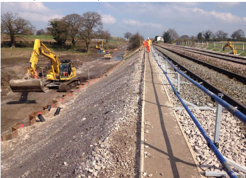
Pictured above: Showing sheet piled wall and embankment regrade in progress.
