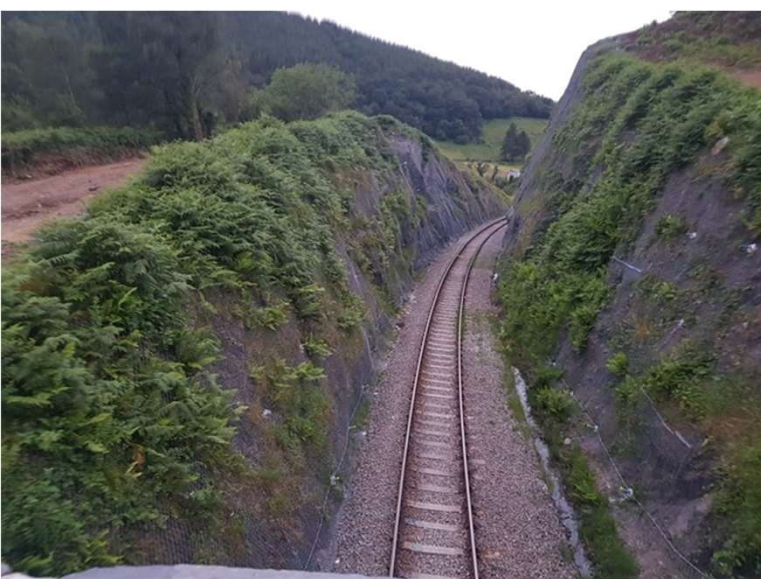
Pictured above: Commins Coch-July 2021- 12 months after works were completed.
