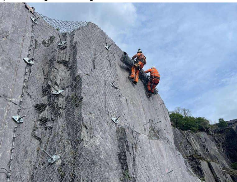
Pictured above: SPIDER rock fall mesh being installed over buttress feature.
