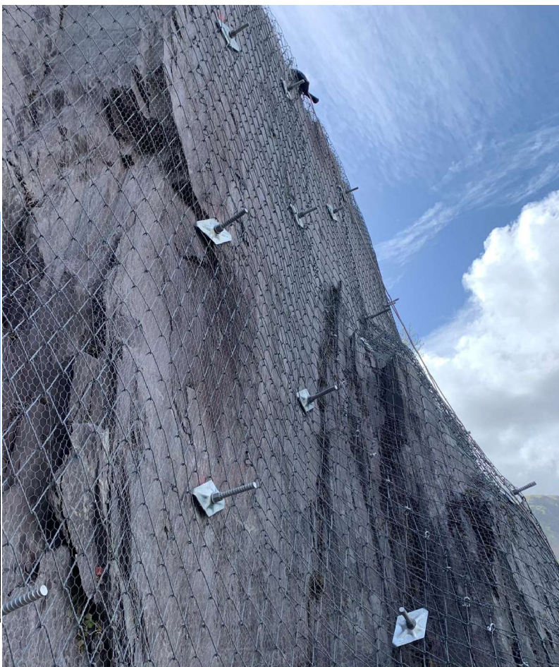
Pictured above: Fig 1) Rock bolts being spun into resin by Rope Access Technicians. Fig 2) Profiled SPIDER mesh.
